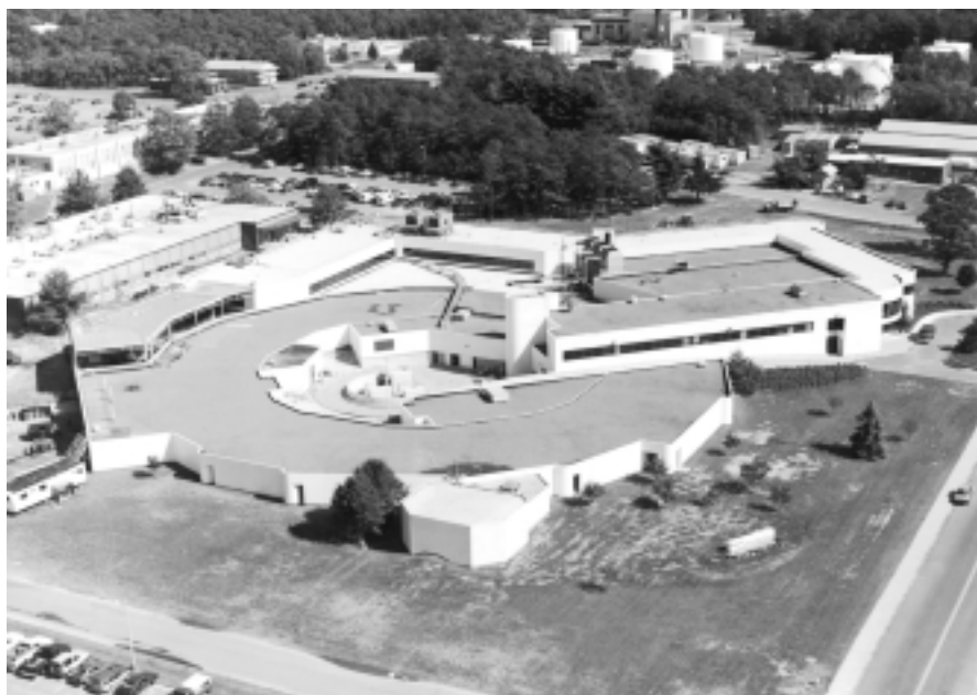
The National Synchrotron Light Source at Brookhaven National Laboratory on Long Island, New York, produces brilliant X-rays, or synchrotron radiation, that can be used to determine the 3-D structure of complex proteins. (Photo courtesy of Brookhaven National Laboratory)
